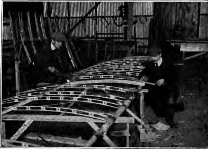
Fig. 31. Assembling the Main Planes of a Bleriot Monoplane
