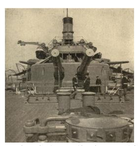
After Deck on the Oregon, Showing Two 13-inch, Four 8-inch, and Two 6-inch Guns.
