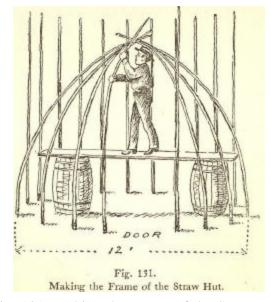
Fig. 131. Making the Frame of the Straw Hut.
